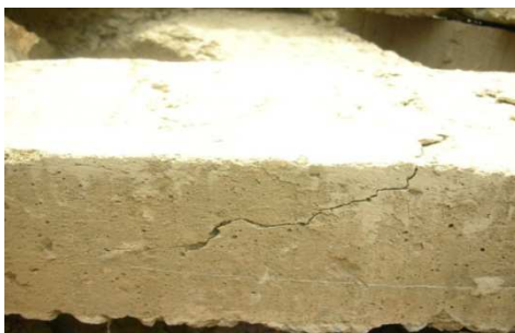
Figure 7. Crack Failure of Beam
