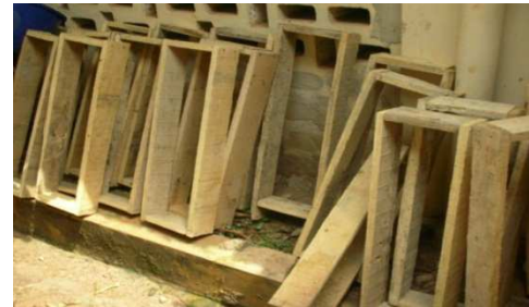
Figure 2. Wooden Formworks
